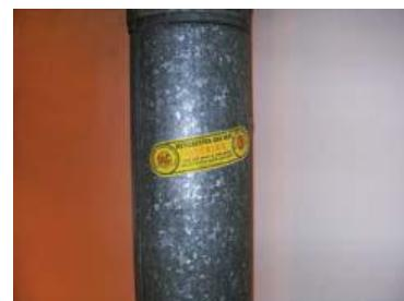
Figure 43 Metal clad gas flue containing chrysotile lining
