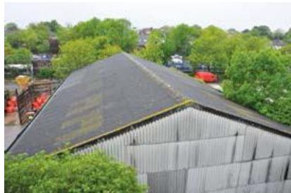
Figure 32 Asbestos cement roof and cladding
