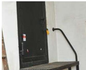
Figure 45 'Durasteel' composite steel and asbestos fire door
