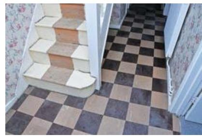
Figure 39 Asbestos-containing vinyl floor tiles
