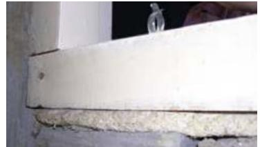
Figure 27 Amosite asbestos rope packing on riser door frame
