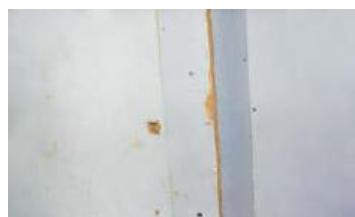
Figure 24 Chrysotile paper on fibreboard boxing
