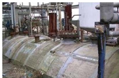
Figure 12 Lagging on large petrochemical vessel
