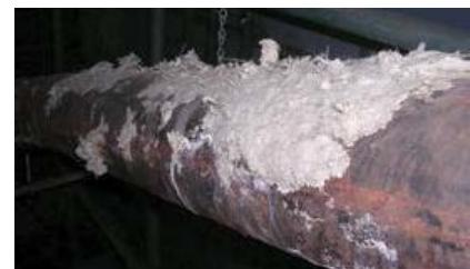
Figure 11 Amosite lagging in very poor condition on steam pipe
