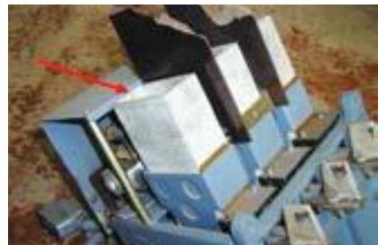
**Figure 49** Electrical switchgear with asbestos flash protection
