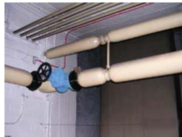
Figure 4 Pipe uncertainty: Top pipe is non-asbestos. All pipes should be sampled
