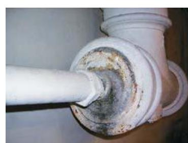
Figure 30 Amosite and chrysotile packing on waste pipes
