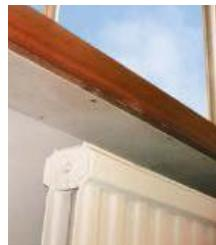
Figure 20 AIB panel between radiator and window
