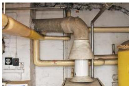
Figure 34 Asbestos cement boiler flue
