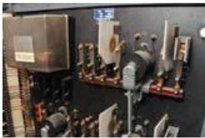
**Figure 50** Open electrical switchboard with asbestos flash guards
