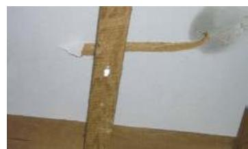
Figure 25 Chrysotile paper on strawboard ceiling panels
