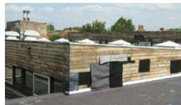
Figure 23 AIB fascia panels with wood effect finish
