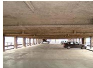
Figure 7 Sprayed limpet on car park roof
