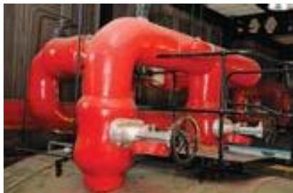
**Figure 48** Asbestos-insulated supply pipes
