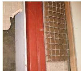
Figure 21 AIB column fire protection in CLASP building
