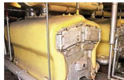
Figure 13 Amosite lagged boiler with hard plastic coating
