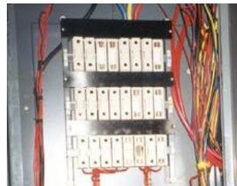
Figure 46 Asbestos tape flash guards in a fuse box
