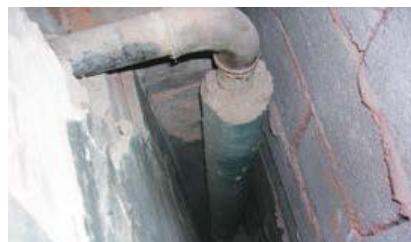
Figure 9 Lagged pipe in wall cavity
