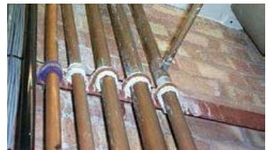
Figure 29 Chrysotile cloth on pipes
