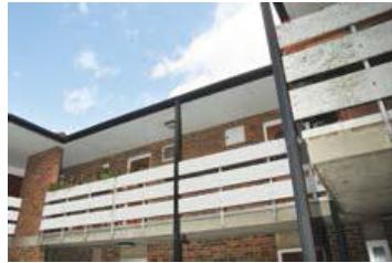
Figure 18 AIB exterior panel on open walkway
