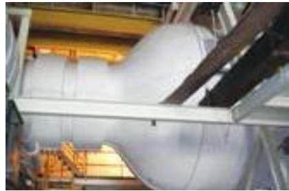
**Figure 51** Vessel clad in amosite insulation
