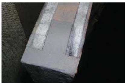
Figure 14 Asbestos panels inside fire door
