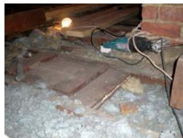
Figure 6 Loose asbestos used as loft insulation
