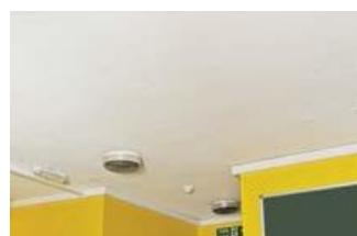
Figure 36 Asbestos textured coating on ceiling
