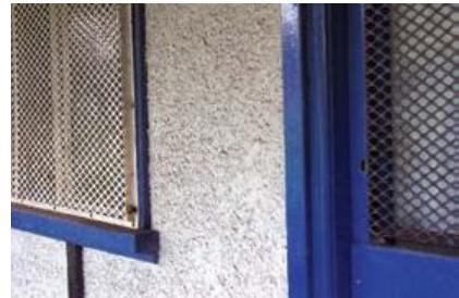
Figure 33 Chrysotile pebble-dash exterior wall coating
