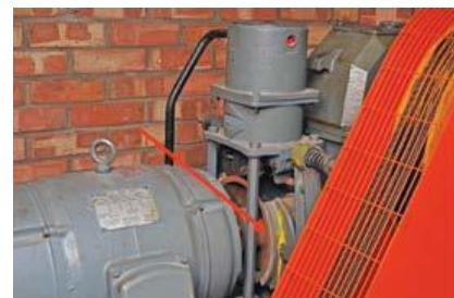
Figure 42 Asbestos brake lining on output shaft of AC motor
