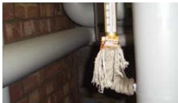
Figure 28 Asbestos rope lagging to boiler thermometer
